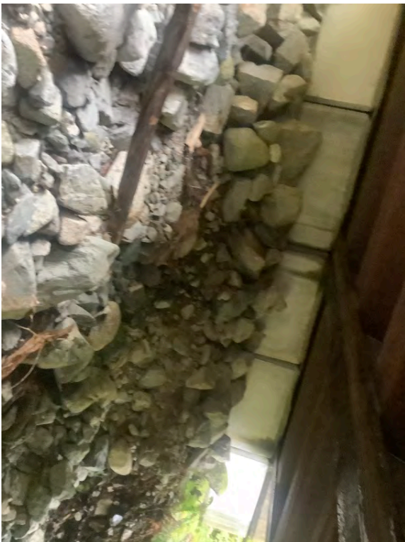
Left Bank Abutment when facing downstream
