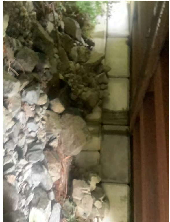
Right Bank Abutment when facing downstream
